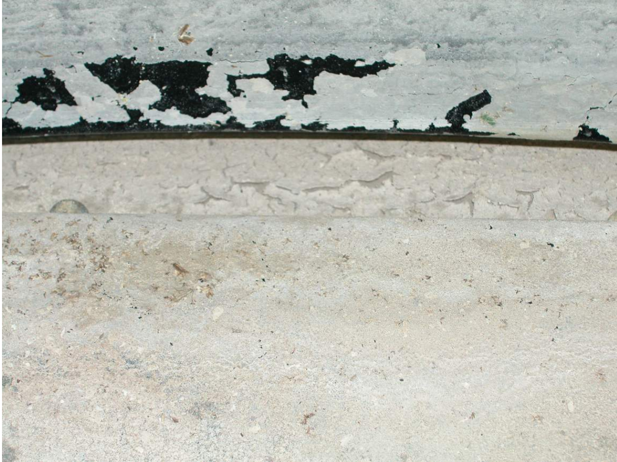
Figure 10. Close up image of scale flaking in Unit #2 basin (Side Stream Filter Only)
